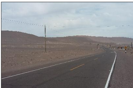
VIA PRINCIPAL CARRETERA PANAMERICANA
